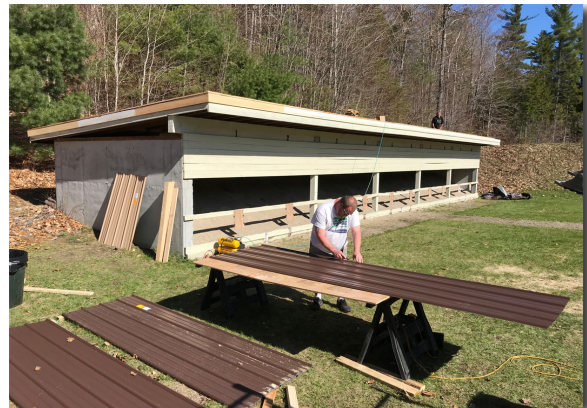
Installation of a new roof at the Owl Brook Hunter Education Center's shooting range.
