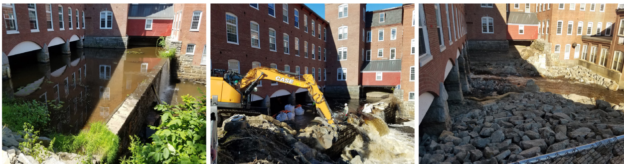
Lower Sawyer Mill Dam, before, during, and after deconstruction.
