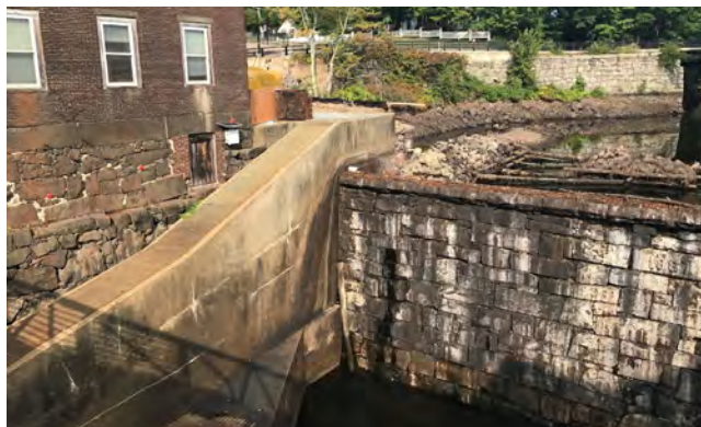
Repairs were made to the dam on the Lamprey River in Newmarket including dam boards, grout holes, and a new shutoff valve.
