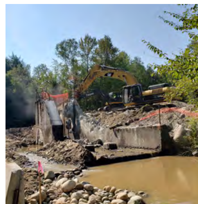
An old dam being removed on the South Branch of the Gale River in Bethlehem to improve habitat for wild brook trout.
