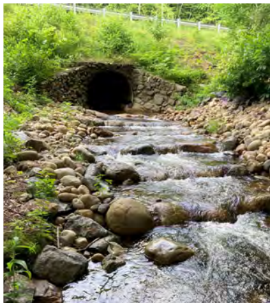
The Department assisted with design and installation a “fish ramp” to improve fish passage at this culvert on Bartlett Brook in Warner.
