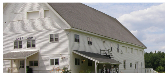
Shea Farm Transitional Housing Unit (C1 & C2)
