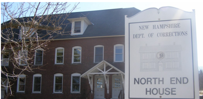
North End Transitional Housing Unit (C1)
