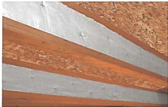
A proprietary ceramic fiber blanket insulation can be attached to the web of the I-joists to comply with IRC provisions. Photo courtesy of Mei Guo International, LLC (USA) FireBreak™.
