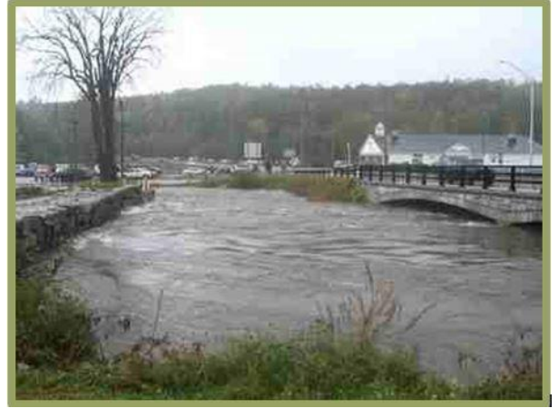
Stone arch bridge threatened by flood
