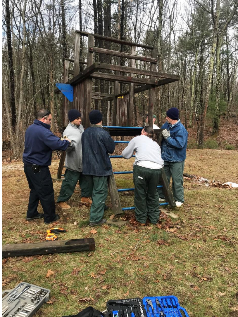
The TWC work crew reassembling the play structure.
