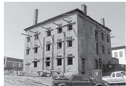
South elevation of the Eagle Block, showing work in progress. (Photograph by James L. Garvin)
