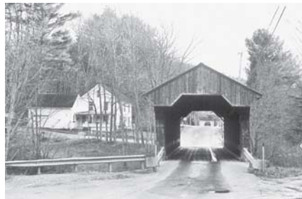
Waterloo Historic District, Warner NH. Listed September 13, 2003. (Photograph by John T. Howe)
