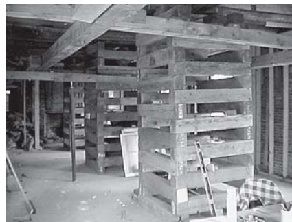
Temporary cribbing, Eagle Block. (Photograph by James L. Garvin)
