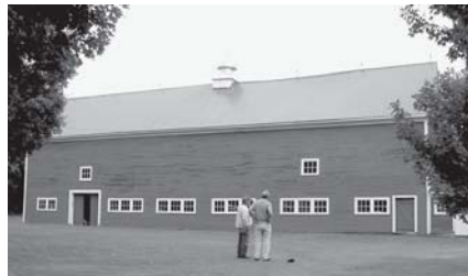
Barn owner Dan Downes and Grant Construction Manager Francis Gilman survey the fine results of this summer's work at Spring Hill Farm in Lebanon. (Photograph by Elizabeth H. Muzzey)
