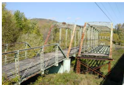
Meadow Bridge as it appears in 2008, with one river span moved to the southern shore of the Androscoggin River and the second river span visible in the distance on the northern shore.
