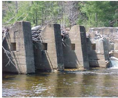
Ruins of concrete buttress dam (1929), Bearcamp River, South Tamworth, NH (Photograph by James L. Garvin)
