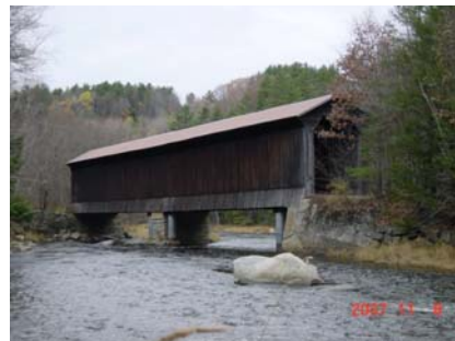
Pier Covered Railroad Bridge (1907) over the Sugar River, Newport, N. H. (Photograph by James. L. Garvin)
