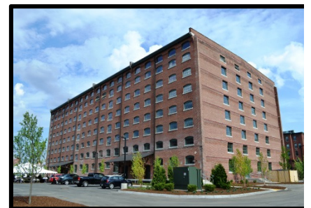
The award-winning rehabilitation of the North Cotton Storehouse , Nashua.
