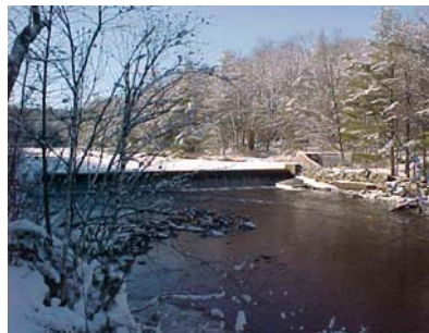
West Henniker Dam, rebuilt in 1936 on the site of dams dating back to the 1700s.
