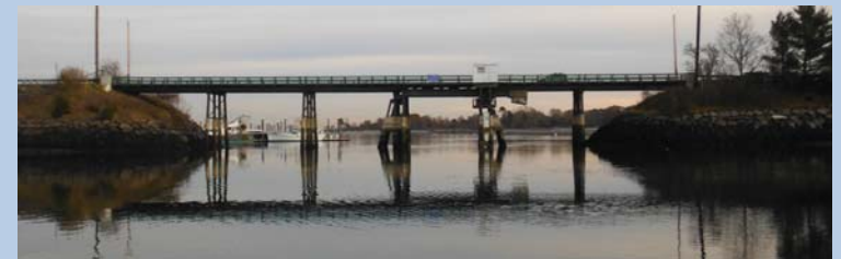
Existing Bridge Looking East
