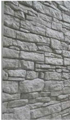
Dry Laid Stone
