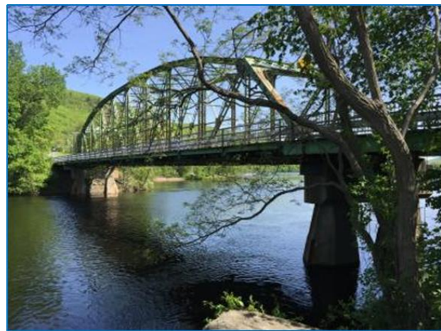
Charles Dana Bridge
