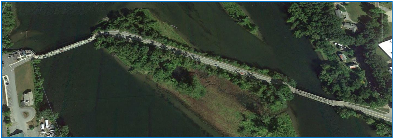
Figure 1 - Anna Hunt Marsh Bridge - Photo Left; Charles Dana Bridge - Photo Right (Looking North / Upstream)
