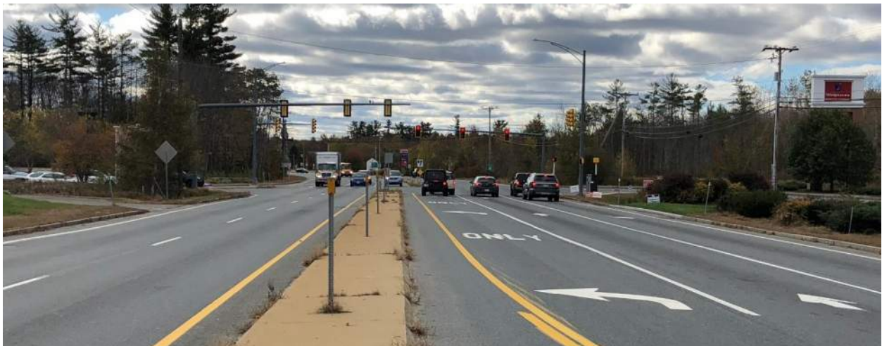
NH Route 125 facing south looking towards Fresh River Road
