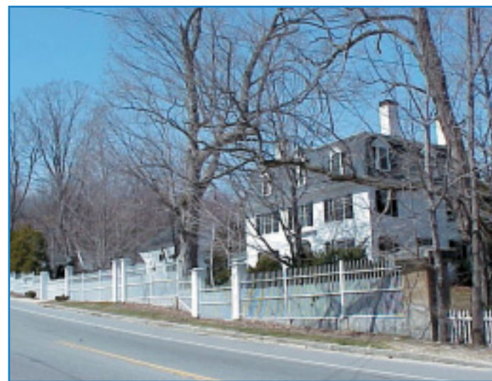
Along Route 124 in New Ipswich, New Hampshire, public input helped shape the landscaping and roadway design in a historic district.
