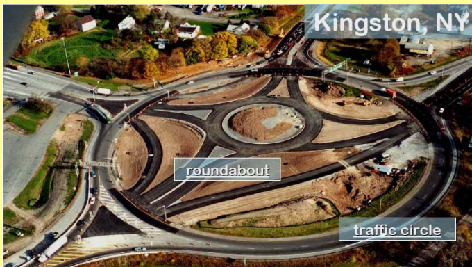
Size – Roundabouts are much smaller than a Traffic Circle. This smaller size makes them safer, slower and more efficient.
