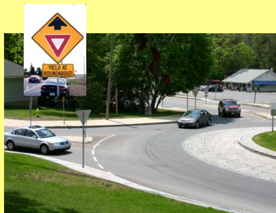
Yield at Entry – Traffic entering a roundabout must yield to traffic already in the roundabout. Many traffic circles do not follow this rule.
