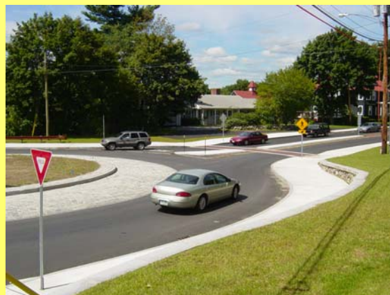
Narrow Lanes – Narrow entry, exit and circulating lanes control vehicle speeds and creates a more uniform speed through the roundabout.
