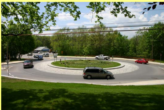
Speed – Because of the smaller circle size in a roundabout, travel speeds are reduced to 15-20 mph. This results in a safer intersection that provides a higher capacity than a traffic circle.
