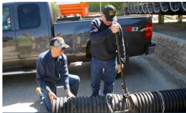
The top innovation for 2013, as decided upon by a panel of judges, was a "pipe puller connector," which was designed and fabricated by District 4's Bob Hebert and Kevin Magoon (PS #404 Hillsborough)
