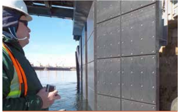
Dave Powelson, Chief of Structures in the Bridge Design Bureau, takes a close-up look at the fender protection system on the Memorial Bridge after it was struck by a tanker ship on March 7th.
