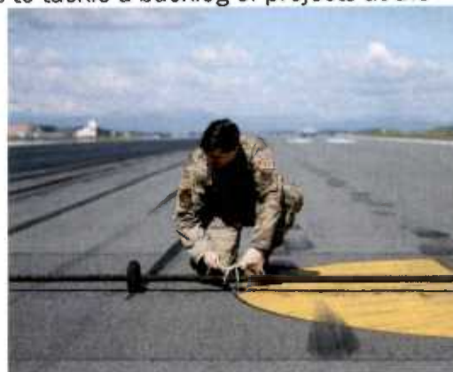
SSgt Carson Lustenberger secures an aircraft arresting system while at Misawa Air Base, Japan.
