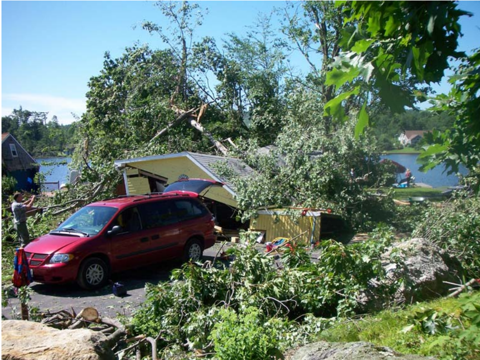
Property damage along Northwood Lake caused by the tornado that struck central New Hampshire last July. N.H. Department of Safety photo
