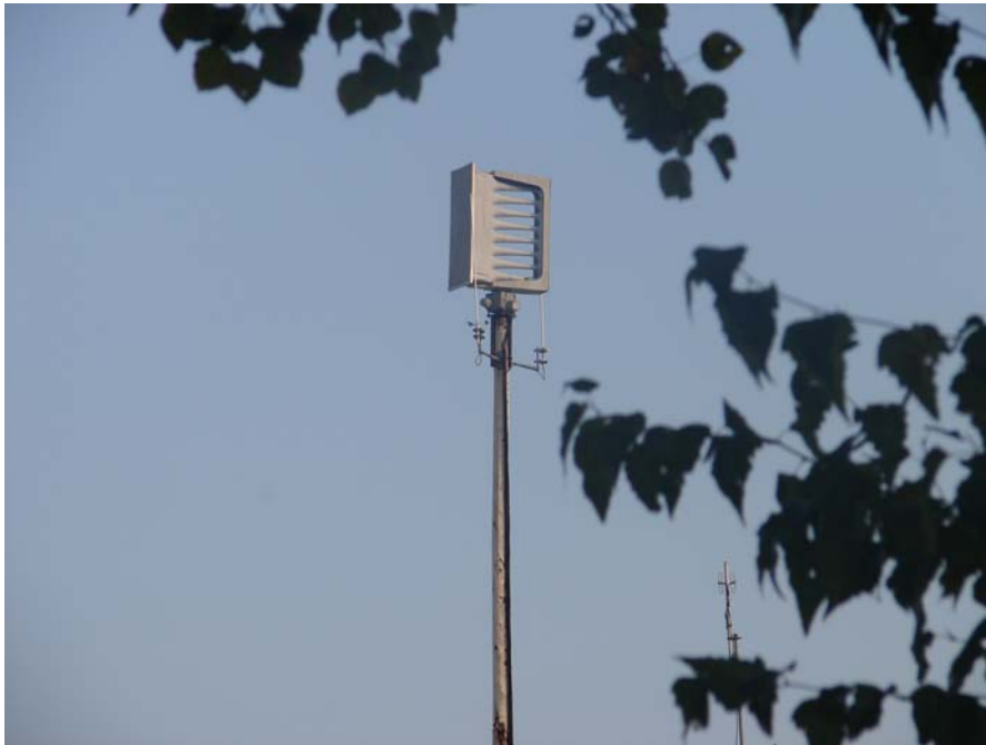
Seabrook emergency siren. Photo courtesy of FPL Seabrook Station.
