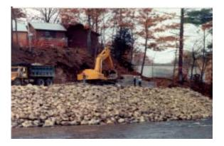
Photos 1 and 2: Before and after pictures of streambank stabilization done under EWP.
