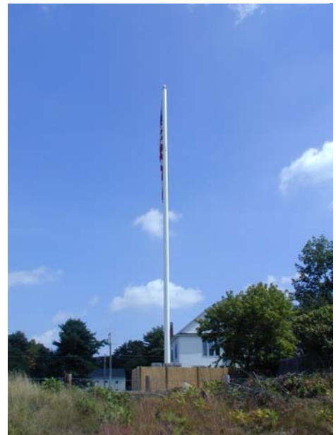
This "flag pole" is also a flush-mounted monopole which is located in Hudson, NH.
