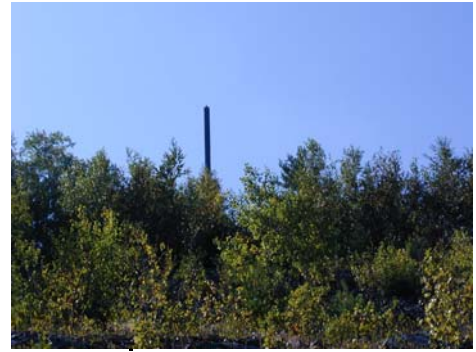
This "brown stick" is a flush-mounted monopole along Route 101 in Raymond, NH.
