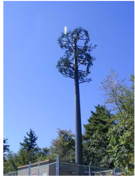
This "stealth tree" facility is located in Dublin, NH and is quite difficult to identify from afar.
