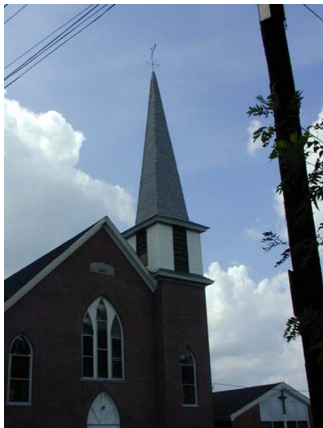
This Hudson church also serves as a telecommunications facility with antennas located in the steeple.
