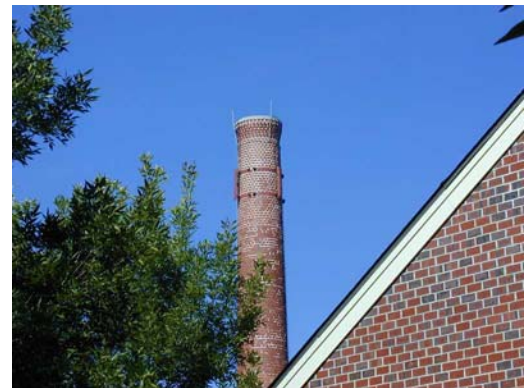
This "chimney mount" is located in Exeter, NH and is practically impossible to detect.
