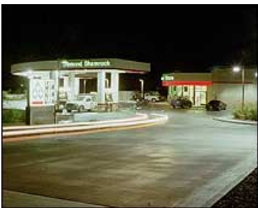
Example of Over-lighting
