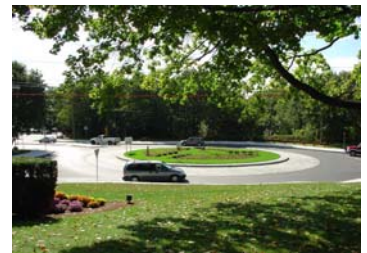
Roundabout in Nashua, NH.
