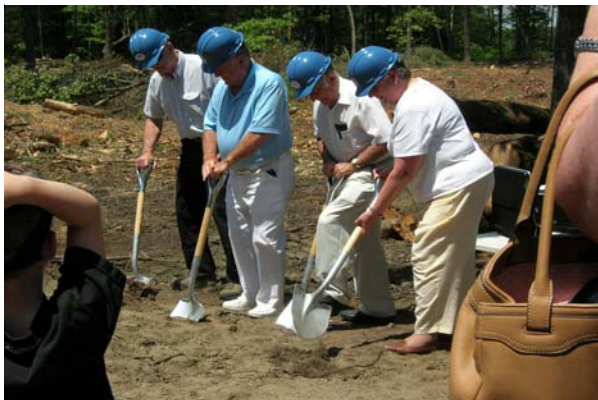
Clerk of the Works, Bernie Manor, Donors: Al Rodgers, Phil Rodgers, Project Administrator Elaine Brody. Groundbreaking for the new George H. and Lila M. Rodgers Memorial Library.
