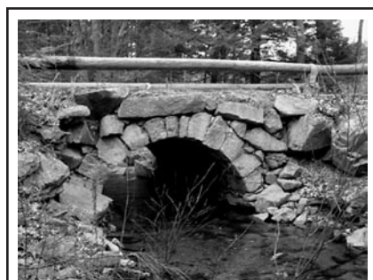
Dry-laid arched culvert, Memorial Highway over Temple Brook, Temple, NH. Photograph by James L. Garvin
