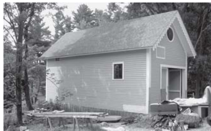
Drainage on this hillside location was a particular dilemma for the Milan Walter Harris Barn project in Harrisville. "Gingerbread" trim on the barn was restored to match details on the house. (Photograph by Elizabeth H. Muzzey)
