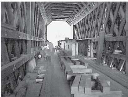
Contoocook Covered Bridge, Interior View. (Photograph by James L. Garvin)
