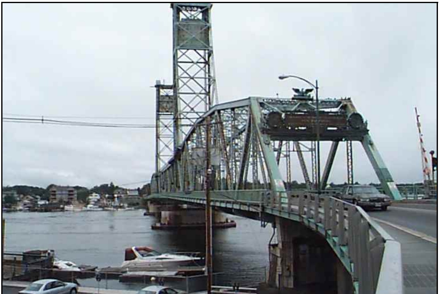
Memorial Bridge – NH approach looking toward Maine
