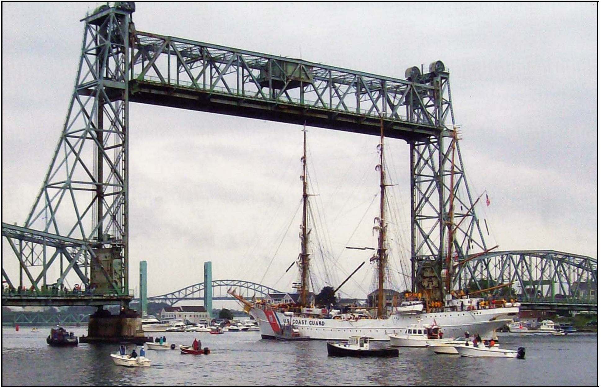
Memorial Bridge – looking north
