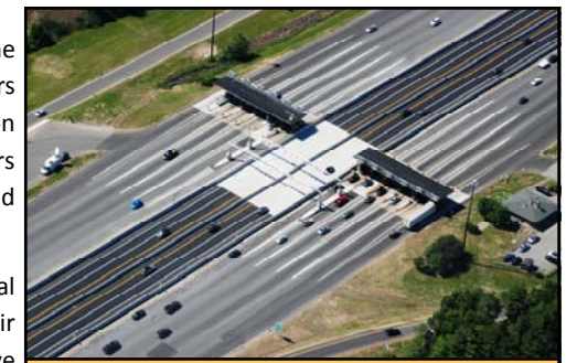
Aerial photo of the new Hampton Toll Plaza Open Road Tolling system on I-95
