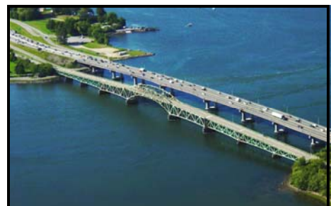
Newington-Dover Little Bay Bridges & Spaulding Turnpike Construction
