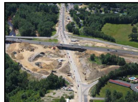
Rochester Spaulding Turnpike Expansion (Exits 11-16)
