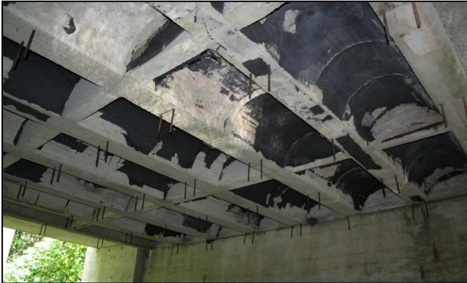
Figure 3.20: Alton 096/287. Tarpaper used between the forms and the concrete shown still adhering to the arches. Note hangar bolts for the forms and concrete diaphragms between the arches encasing the beam tie-rods. Survey Photo July 2010.
