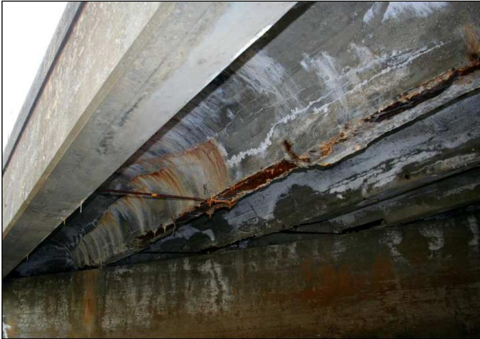
Figure 4.5: Newbury 120/078 [1936?]. Severe cracking and spalling of concrete encasement and rusting of I-beams. RMC Photo April 2009.
